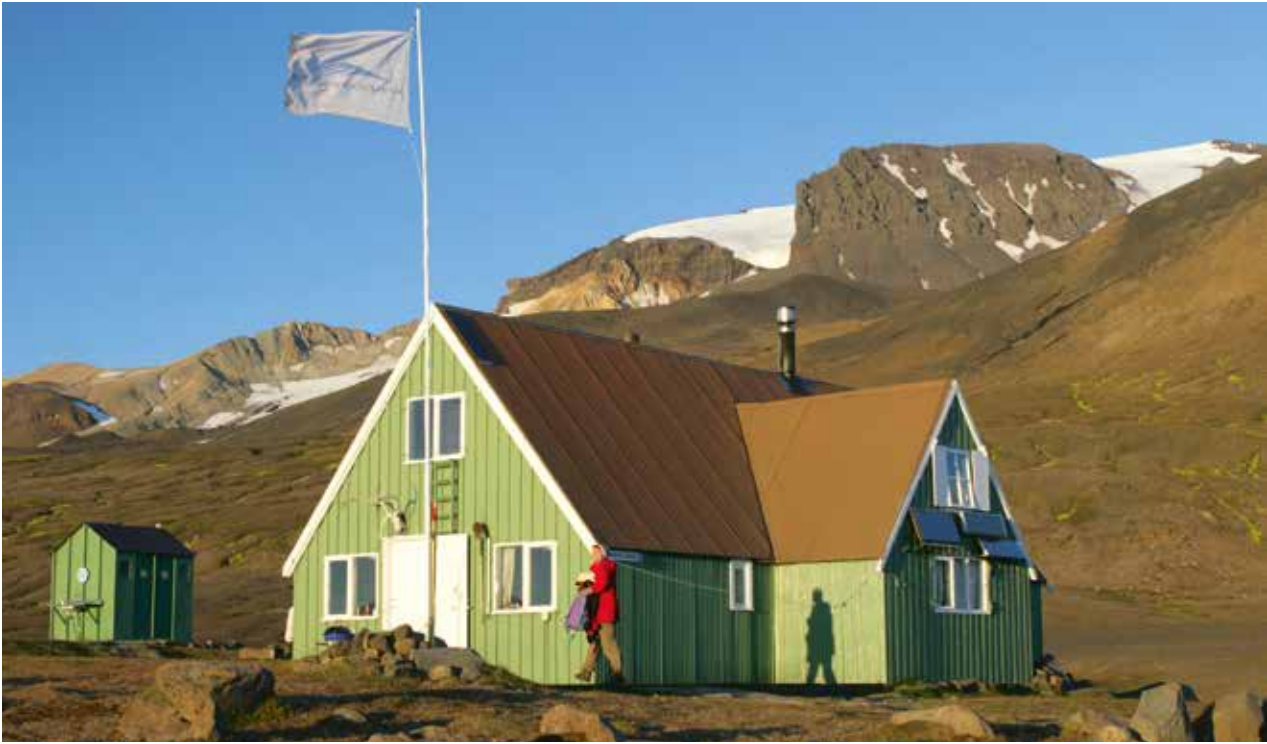
Examples of infrastructure within Vatnajökull National Park. Top: The overnight hut at Snæfell © Skarphéðinn Þórisson. Middle: The research hut of the Glaciological Society at Grímsfjall on Vatnajökull ice cap © Snorri Baldursson. Bottom: Gamlabúð visitor centre at Höfn in Hornafjörður © Helga Davids.
