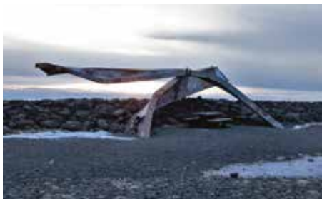
Top: The bridge over Heinabergsvötn was built in the 1940s, but shortly afterwards the river moved to the west © Snævarr Guðmundsson. Bottom: The remains of the Gígja bridge stand now as a memorial to the 1996 Gjálp jökulhlaup, 30 December 2017 © Hrafnhildur Ævarsdóttir.
